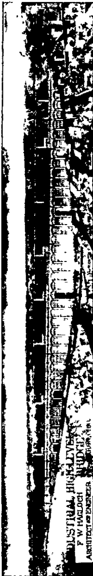
Proposed North Hill Viaduct—Length 2580 ft —Height 98 ft —Width 60 ft —Roadway Overhead—Factories Underneath
